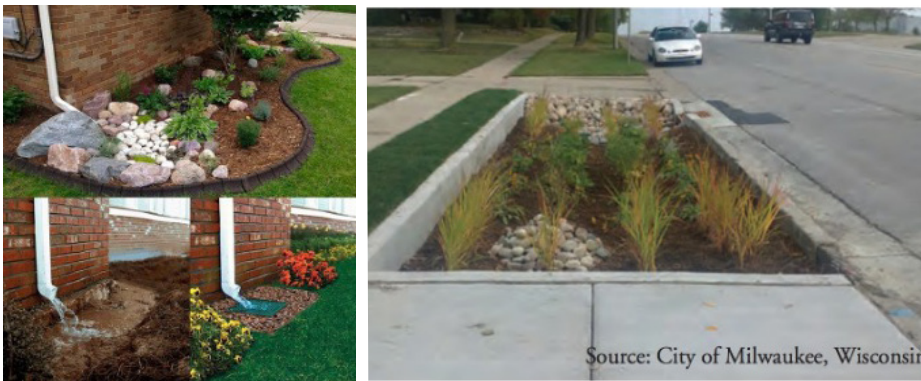
Figure 2.5, top left: The photo collage displays an example of adding rock and vegetation (top) or a dry well (bottom right) below the downspout to prevent runoff. 73 Retrieved from Pinterest.
